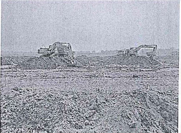
Figure 7 Ash discharge from pond area for low lying area filling
